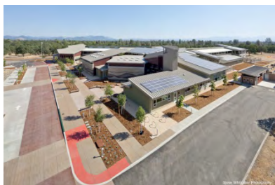
Figure 22. Redding School of the Arts Powered by PV and Wind Energy. Source: http://www.solar-design.com/SDA-Today/renewable-energy-serves-redding-school-of-the-arts/?toperStarEhJUS=1
