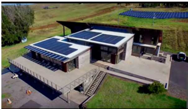
Figure 16. Utilize the site and building’s roof to generate renewable energy through photovoltaic. Source: http://www.hpa.edu/academics/energylab
