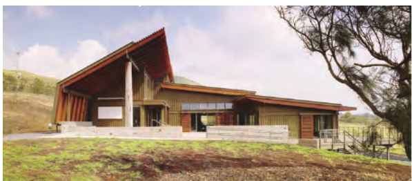
Figure 15. A traditional “Tropical Three Pitch Roof” design features a shaded lanai facing south. Source: http://www.hpa.edu/academics/energylab
