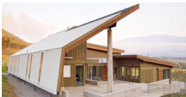
Figure 20. The south-facing outdoor classroom is supported by a salvaged native ohia wood column. Source: Institute, 2019.
