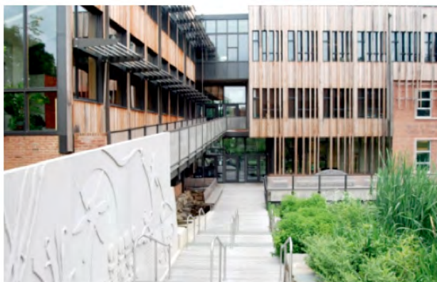
Figure 13. The building's "skin" is made from reclaimed wine casks. The decking wood came from pilings from the Baltimore Harbor. Source: http://www.sidwell.edu/middle_school/ms-green-building/index.aspx
