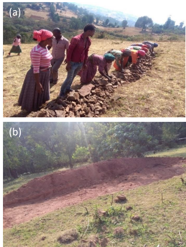
Figure 9. Stone bund (a) and Soil bund (b)
