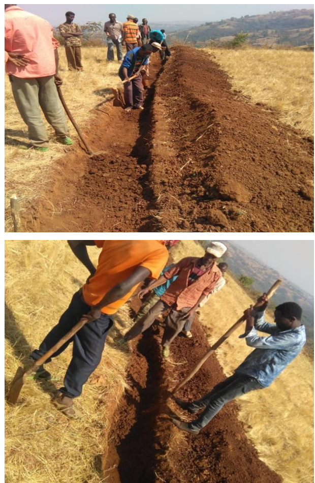
Figure 7. Terracing activity in the study area (Source: Field photo, 2023)
