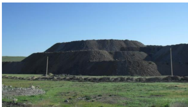
Figure 3 Mining activity resulted in the formation of dumps generally characterized by three tilted strata showing a slope ranging around 60-70^{\circ} .
