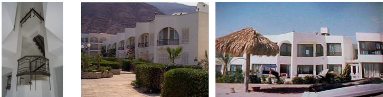
Figure 1. Biogeometrical architecture; architect selection for angles and colors to achieve a balance in energy within the spaces (left)- tourist village in Ain Sokhna from inside and outside the units, (right)- the tourist village in Hurghada, architect: Ibrahim Karim ( www.biogeometry.com ).
