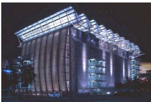
Figure 6. The British Pavilion in Expo, Arch. Grim Shaw- The building shows light structural elements designed from light steel and glass to resist the hot summer climate, as well as the installation of photovoltaic panels on the building, the huge water wall in the eastern side of the building and pass down through the wall painted in a water bath to form a trench around ( https://grimshaw.global/projects/british-pavilion-expo/ ).
