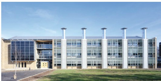
Figure 8b. Environmental response and smart spaces, The Building Research Establishment (BRE) Office Building, shows the solar chimneys and details of the solar station as well as solar fenders moving aesthetic dimension (DeKay and Brown, 2001).
