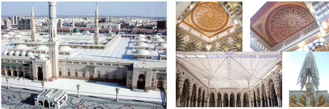
Figure 8a. In the Prophet's Mosque in Madinah domes and electronic tents control and interacting with environmental variables, especially with regard to building technology integrated with the environment, especially with regard to building materials suitable for the hot dry climate, represented by the material Teflon manufactured from tents.
