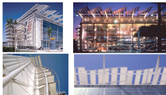
Figure 6. The British Pavilion in Expo, Arch. Grim Shaw- The building shows light structural elements designed from light steel and glass to resist the hot summer climate, as well as the installation of photovoltaic panels on the building, the huge water wall in the eastern side of the building and pass down through the wall painted in a water bath to form a trench around ( https://grimshaw.global/projects/british-pavilion-expo/ ).
